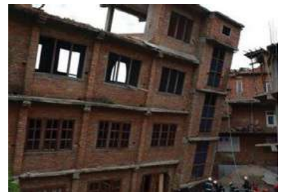
फोटो : Tilting Building by Gorkha Earthquake 2072
