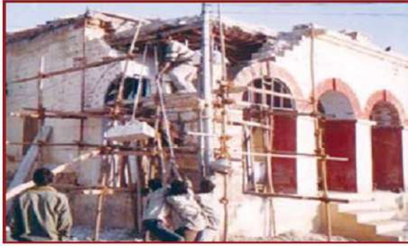
Cracked arcade being restored stone by stone
