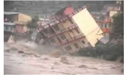
फोटो : Building swept away by Flood
