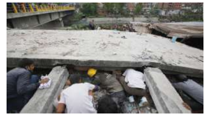
फोटो : Building Colapse due to weak beam column connection in Gorkha Earthquake
