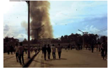
फोटो : Fire at Historical Singha Durbar Building
