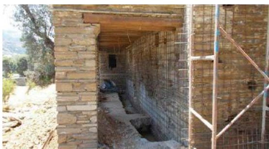
Jacking in Stone Masonry load bearing building
