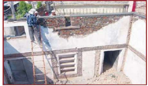
Damaged brick masonry wall being rebuilt to reinstall Rc slab on it
